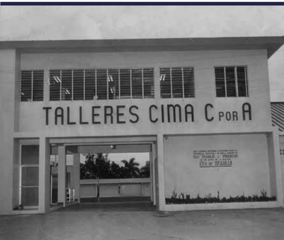
Photo 5: Former business at building site, Santo Domingo 1950
